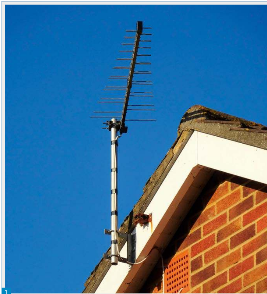
Fig. 1: A small domestic TV antenna mounted on a fascia. Fig. 2: Using a chimney to support a rotator and VHF antennas. Fig. 3: A VHF and UHF antenna mounted on a gable end wall. Fig. 4: A common arrangement for fixing a pole to a brick wall. Fig. 5: One way to keep a wire antenna under tension when supported by a tree.
